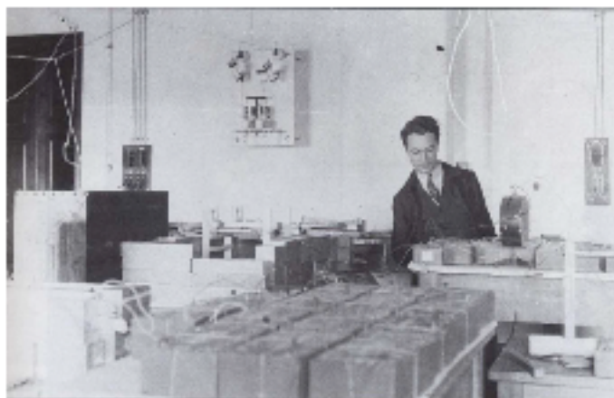
Fig. 1. Bruno Rossi in his laboratory at the Physics Institute of the University of Florence, ca. 1930. To his right are Geiger counters; in front are the batteries with which he powered them. (Rossi family collection.)
